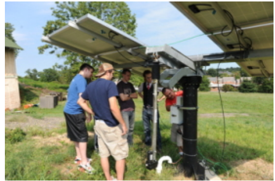
Engineering students install solar panels at DC Franciscan
