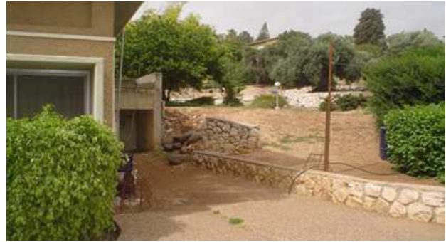
Figure 25: The central area with a dining hall not in use; repairs needed in the retaining wall are delayed (Kibbutz Tel-Yosef, 2010)
