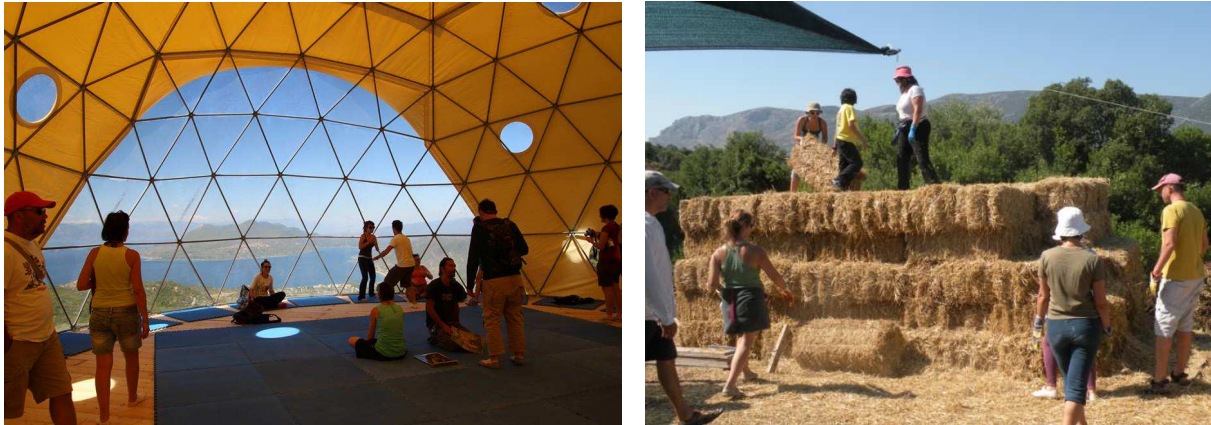
Fig 5. A recently completed large geodesic dome to serve as a common space for various functions at Telaithrion and a strawbale workshop to produce a guesthouse at Elpidohori.
