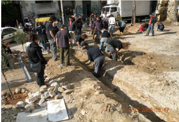
Fig 3a. 1st day of works at the Navarinou Park (3/3/2009)
