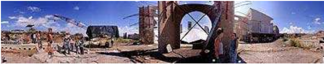
Arcosanti: East Crescent under construction, 1999
